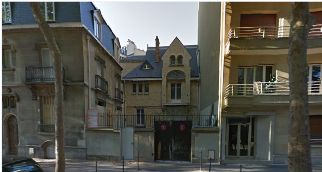
Rue Molitor, Paris
